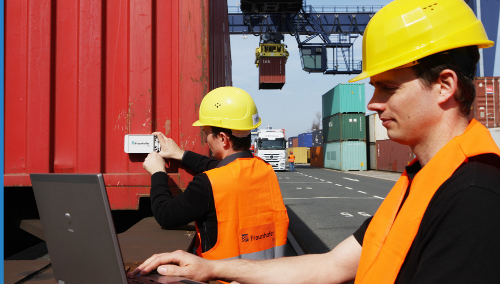
Figure 1: Installation of tracking modules with Energy Harvesting power supply on railway containers
