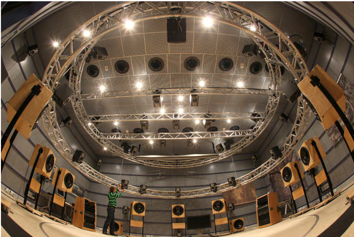
Figure 3: Main reproduction and listening test room Mozart with the set-up of 9 main loudspeakers, 2 subwoofers, and 43 loudspeakers on the walls and the two circular trusses.
